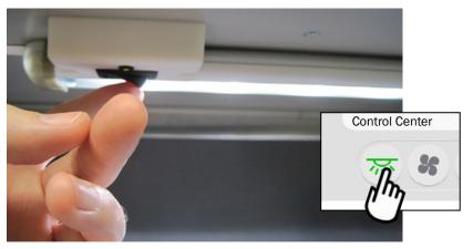
Some cabinets feature task lights with localized switches, while others include a rocker switch in a three-way lighting circuit. With this feature, you can turn the operatory task lights on or off from any cabinet in the circuit. This works the same way when combined with the control center touchscreen. You can turn all task lights on or off via the touchscreen or the rocker switch.
